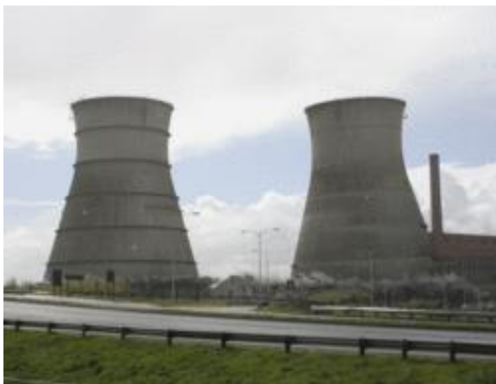
Figure 9. Demolition of the cooling towers of a power station, Athlone, Cape Town, South Africa, 2010
